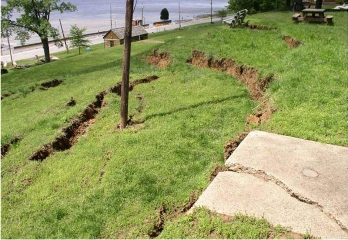
*Figure 75. Newburgh landslide prior to mitigation*
